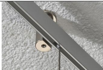
Top support with washer, aluminium track, ø1,5 mm 49 strand stainless steel cable
